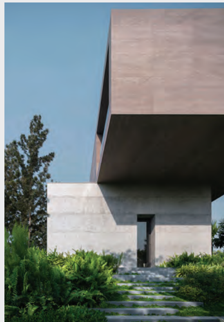
Steps were integrated into green landform, leading to the Party Lawn and Tea Court.
